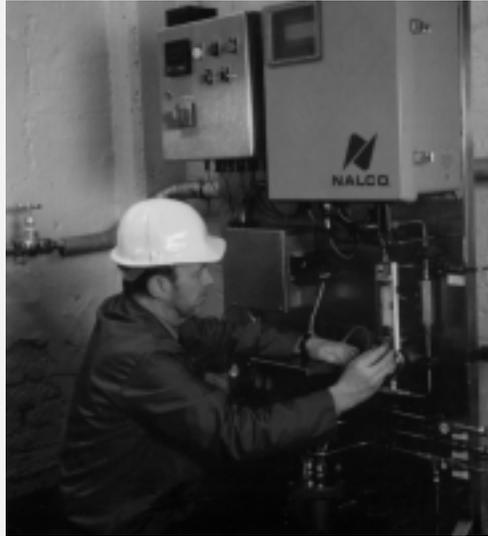
Figure 1: Checking water treatment control system.
