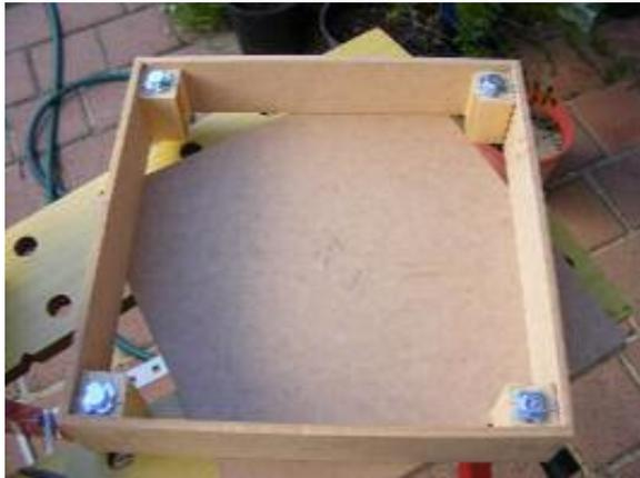
In this picture you can see the basic box outline coming together. If you put the leg tops the same height as the top you can use this to nail the top securely together. The adjustable feet should sit inside the box as shown just below the base. This will also bring the adjustable feet just below the base so they will be ready if required to be used for leveling up. Glue and nail the other two panels so the box takes shape.
